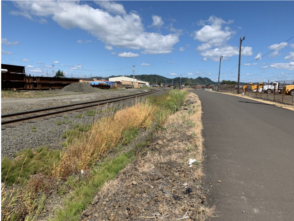
Photo 11: Overview of Wetland 6. Photo taken facing east.
