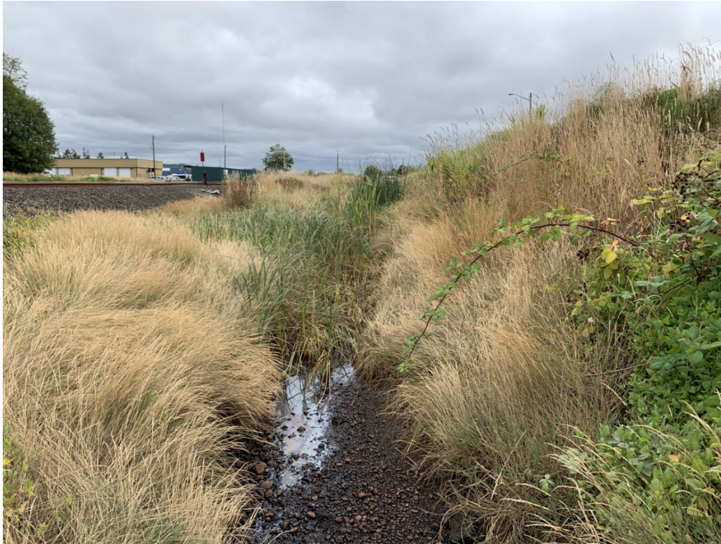
Photo 17: Overview of Wetland 9. Photo taken facing east.
