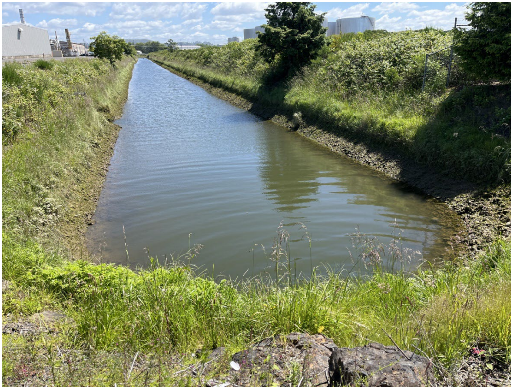
Photo 18: Overview of Fry Creek, north of the culvert. Photo taken facing north.
