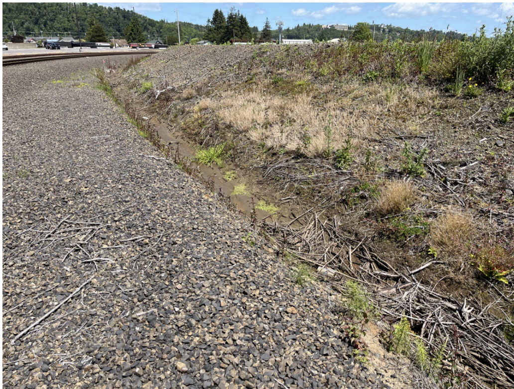
Photo 22: Overview of Ditch 1. Photo taken facing northwest.
